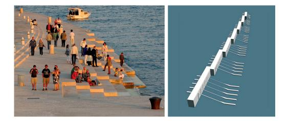
Figure 1: Photo of the Sea Organ in Zadar and a 3D model of the organ pipe system (Bašić Stelluti and Mattioni, 2011)
