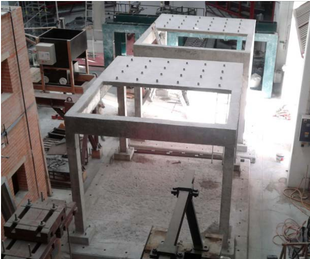
Figure 1. General view of the frame after formwork removal [16].
