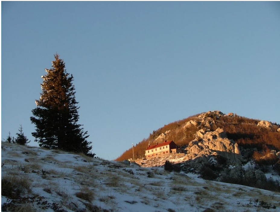
Fig. 4-8. Meteorological station at Vučjak.
