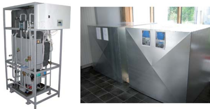
Figure 7.4 Absorption chiller and phase change materials (PCM) latent storage tank for solar cooling and heating, ZAE Bayern, Germany [13] and [26].
