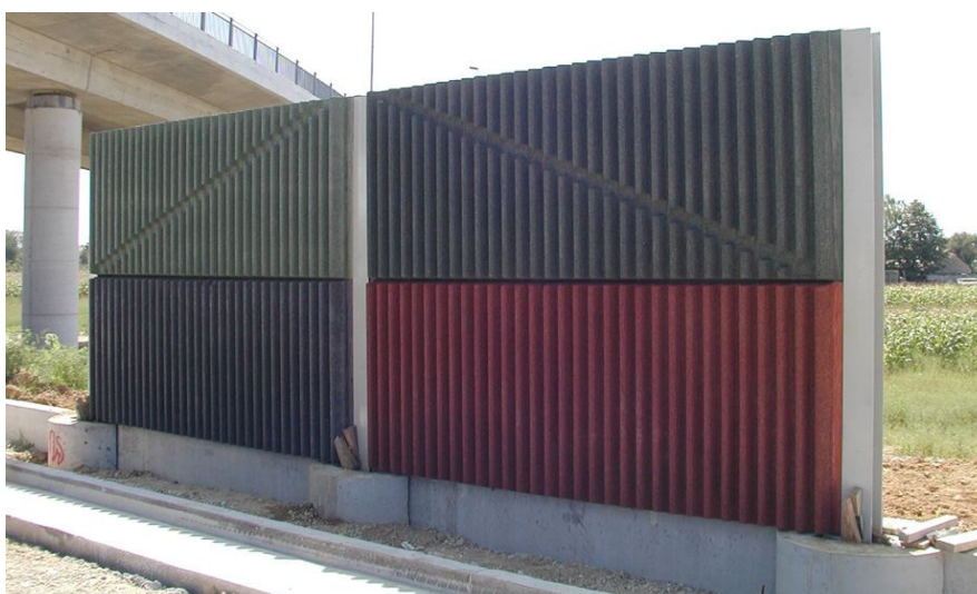
Figure 1. Profiled surface of sound absorbing concrete noise barrier
