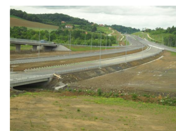
Highway construction in Republic Srpska
