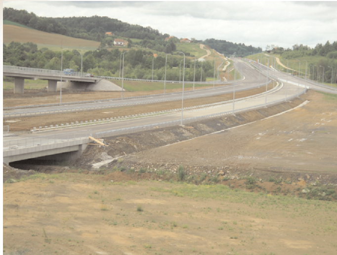
Figure 38: Section of new highway Banja Luka - Gradiška
