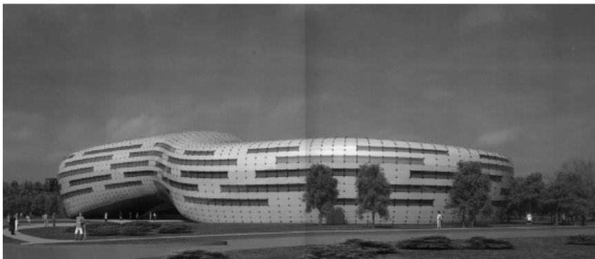
Figure 2. St. Catherine Specialist Hospital in Stubičke Toplice
