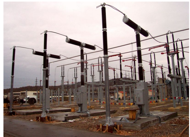
Figure 2: 400 kV switchgear
