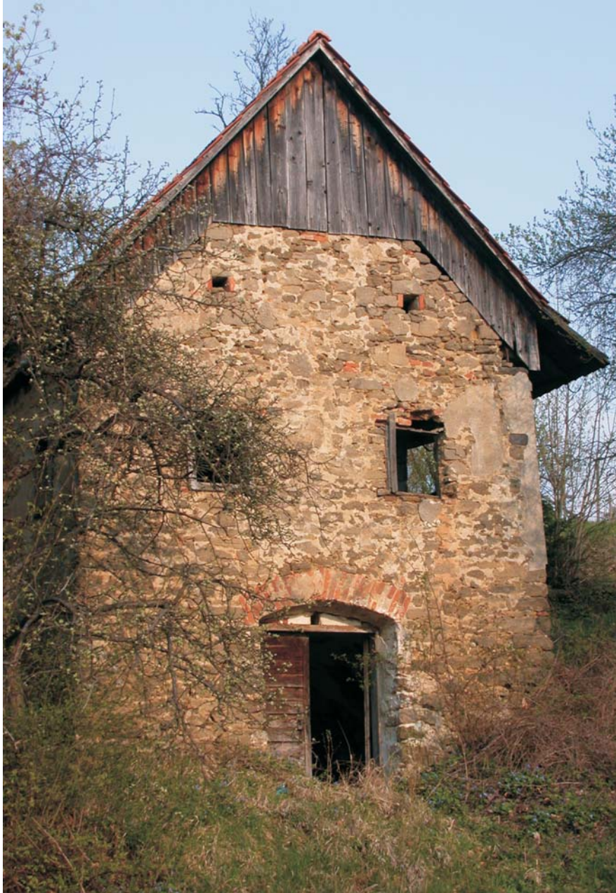
Old building at Beistein.
