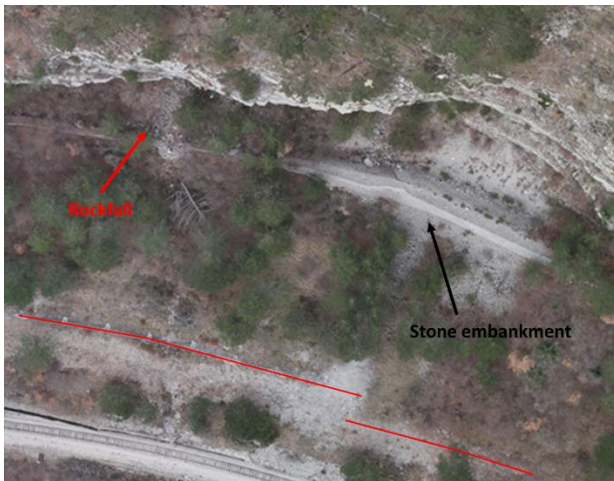
Figure 7. Digital orthophoto map of the western part of the Raspadalica Cliff. On the left side (red arrow) is location of the rockfall occurred on 16 December 2013 that destroyed stone masonry wall; on the right side (black arrow) part of stone embankment. Red lines are rockfall barriers installed above the railway facilities.
