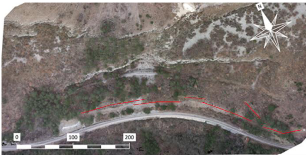
Figure 8. Locations of installed rockfall barriers (red lines) below the Raspadalica Cliff at the digital orthophoto map.
