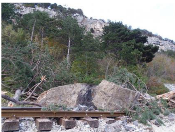
Figure 2. Photo of the rockfall originated from the Raspadalica Cliff on 16 December 2013 (Udovič et al., 2021).
