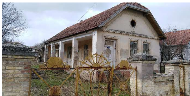
Figure 1. Traditional rammed earth house in eastern Croatia
