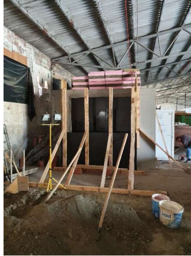
Fig. 4. Formwork assembled before building the wall
