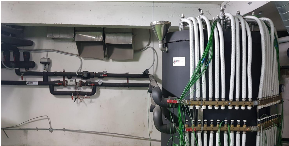
Fig. 3: LTES and flow and temperature control system
