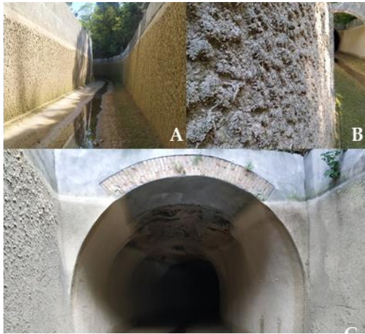
Figure 3: (A) Lateral sides of tufa tunnel; (B) formed tufa; (C) parts of tunnel in dark.
