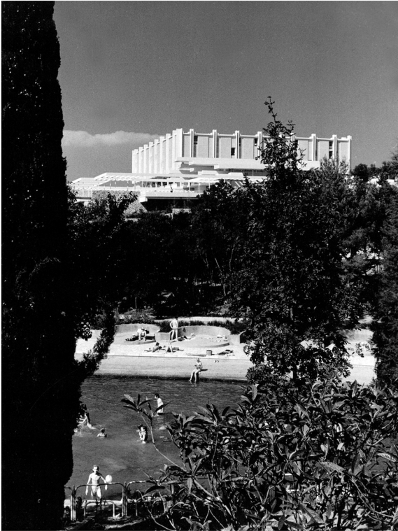
Figure 1: Open-air pool of the main hotel, view from Hotel Palace. Source: Private collection of the Magaš family, Rijeka, Croatia.
