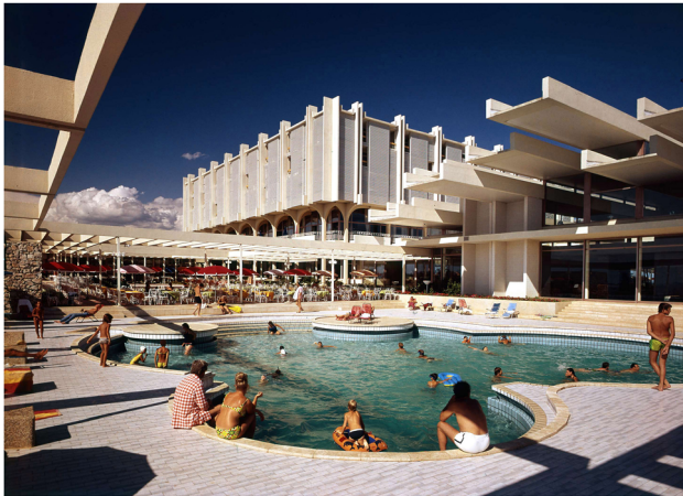
Figure 2: Hotel Palace, indoor and outdoor pools.
