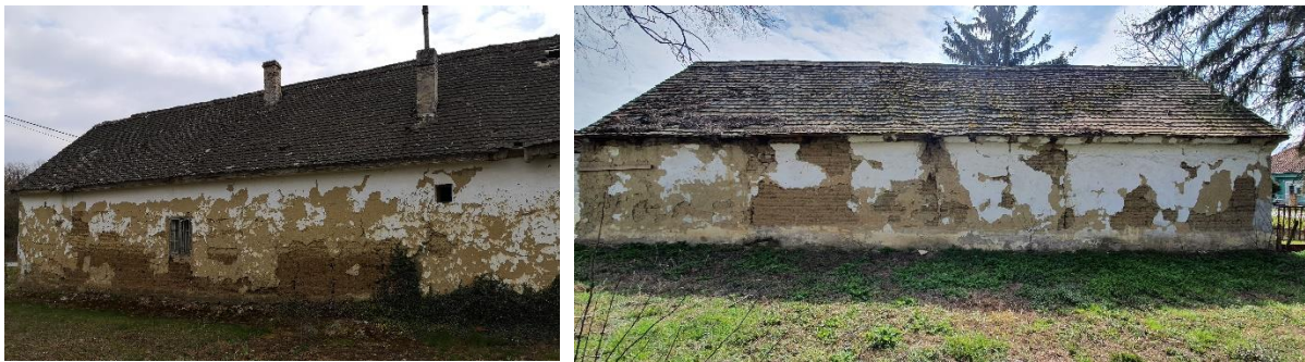
Figure 2. Rammed earth houses in Eastern Croatia (author's archive).
