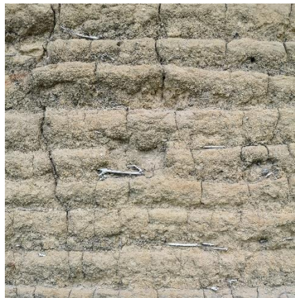
Figure 1. Visible layers on face of the RE wall (author's archive).
