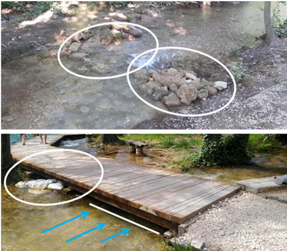
Figure 21. Examples of negative anthropogenic influences (path construction and gravel accumulation) on the hydrodynamics of travertine watercourses.
