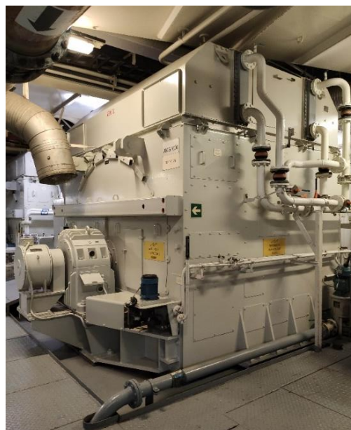
Figure 1: Synchronous generator
