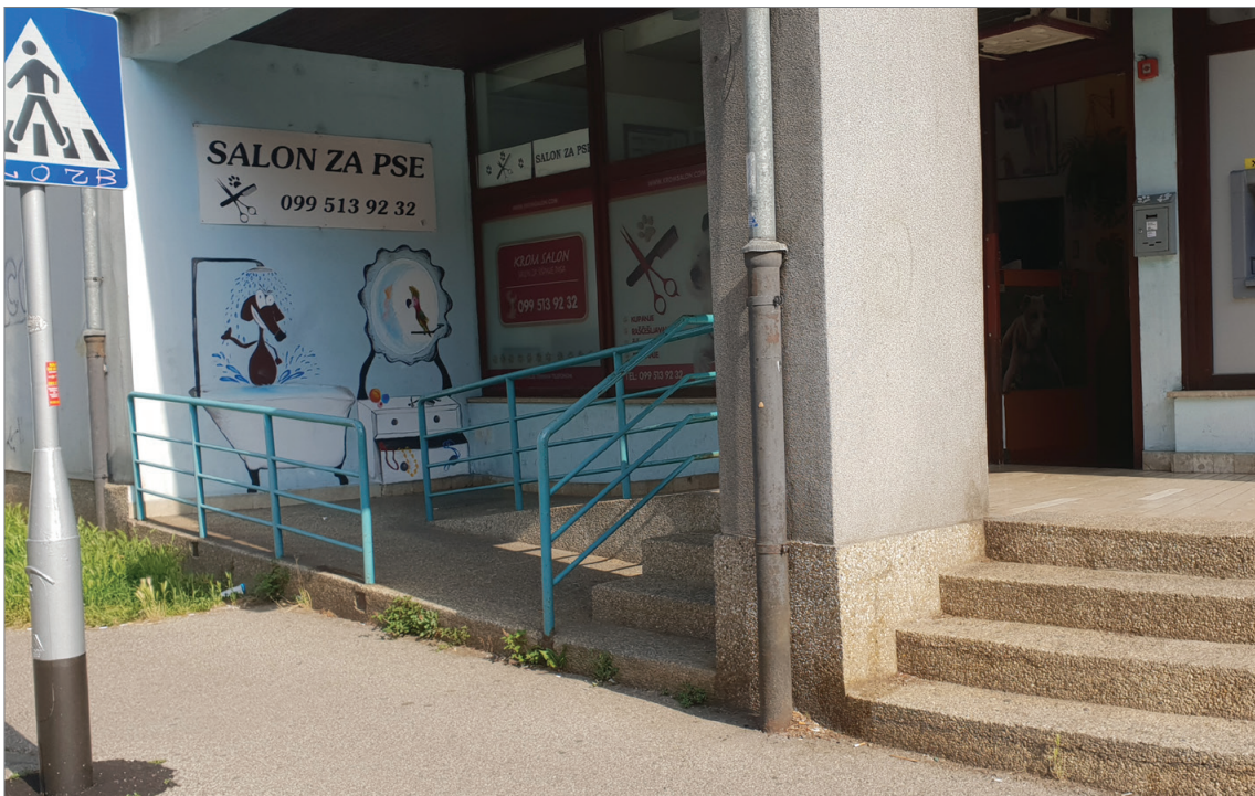
Sl. 10. Primjer otežana prolaska invalidskim kolicima zbog stepenice na kraju rampe Fig. 10 An example of ramp ending in a single stair, complicated to navigate in wheelchairs Snimila / Photo by Andrijana Horvat (2018.)
