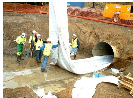
Figure 3: The cured in place pipe process [25] Figure 4: CIPP large diameter liner [26]
