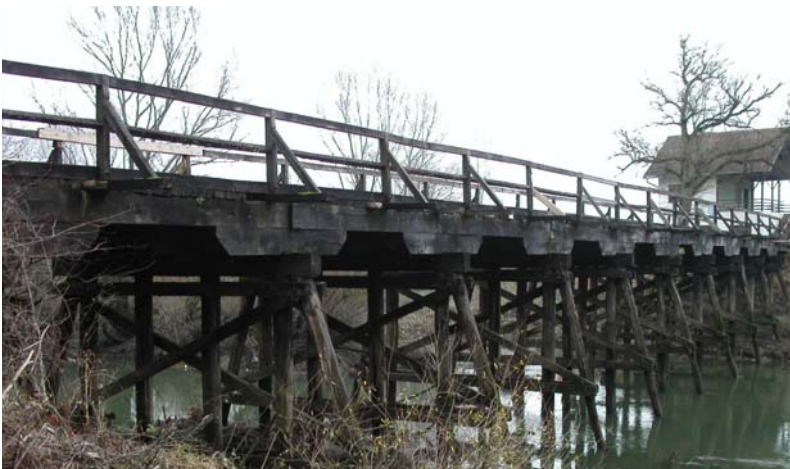
Photo 1. An old timber bridge across the Odra river
