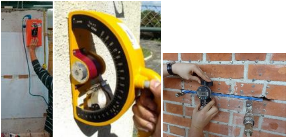
Fig. 2 (left) Ground penetrating radar [14]; (middle) Pendulum rebound hammer [22]; (right) The flat jack test [23]
